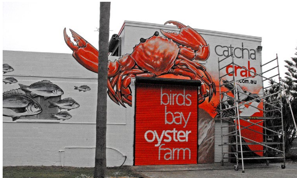
Installing the murals and painting the building exterior
