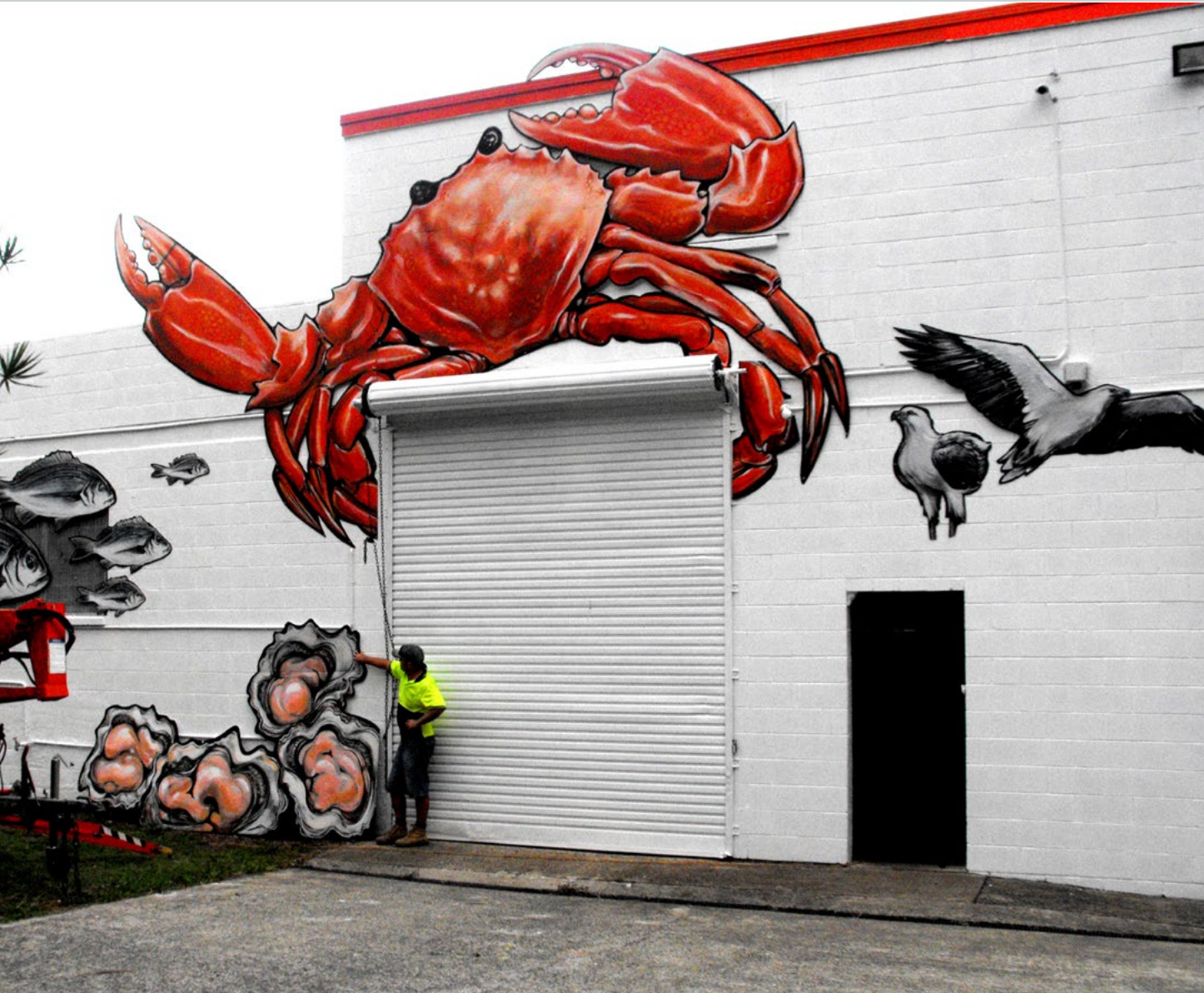
Installing the murals on the building exterior
