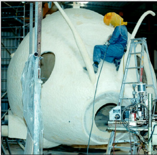
Stage 3 - Building the Head
