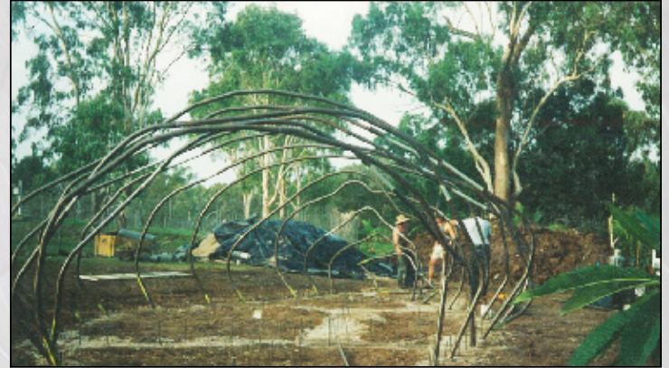
Creating the Armature - additional framing added
