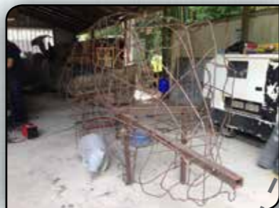
Internal Steel Armature
