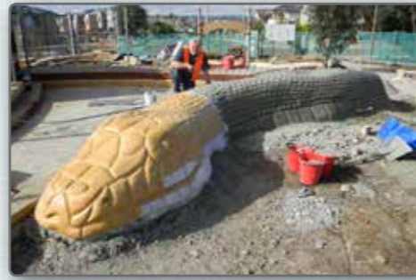
Image 3 - First Coat of Paint being applied
