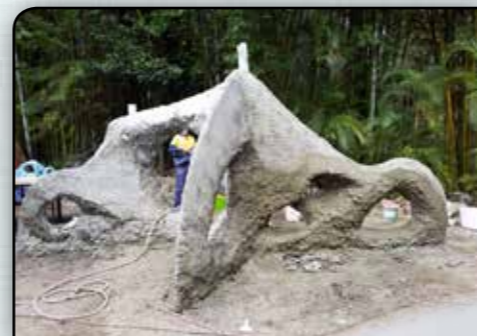
Concrete over mesh
