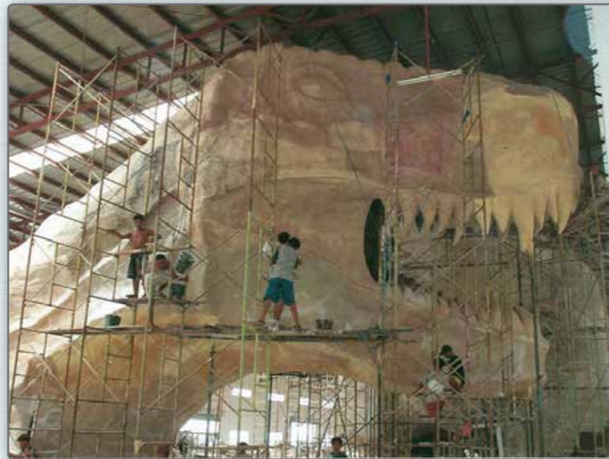
Stage 2 - Scaffolding Around the Head & Neck
