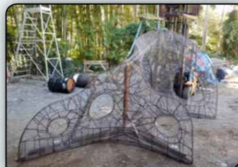
Steel Armature with mesh
