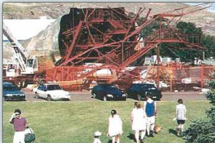
Stage 4 Installation - Inside Steel Armature
