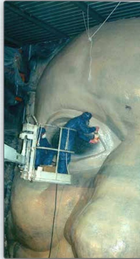
Stage 2 - Sculpting the Eye showing men working from Boom lift. - Note the enormous size of this entry statement.
