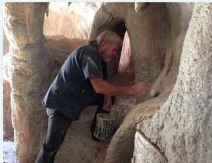
Touching up paintwork seams during installation
