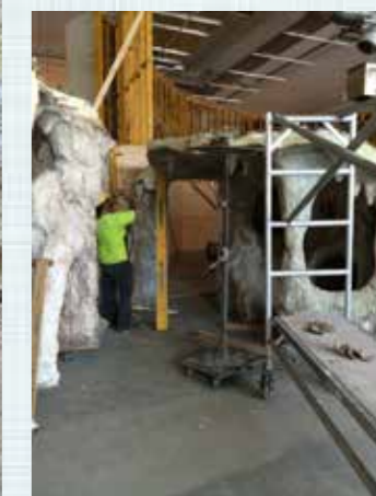
Installtion of Cave
