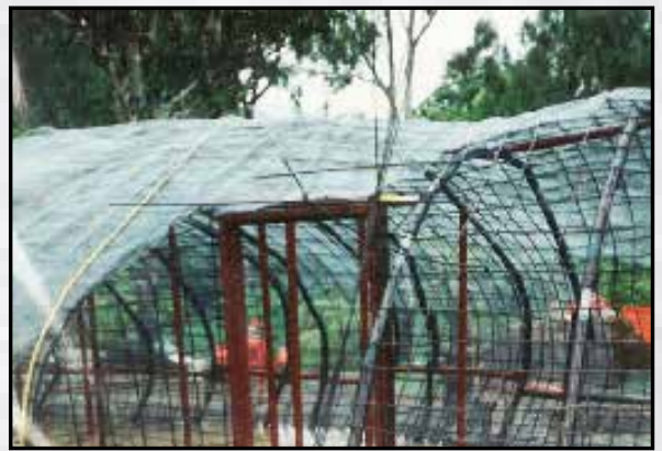
Adding the door frames & application of wire netting over 10mm mild steel bar armature, Necessary for a concrete finish
