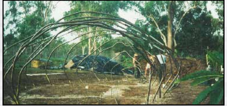
Creating the Armature - additional framing added
