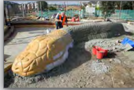
First Coat of Paint being applied - - Image 3
