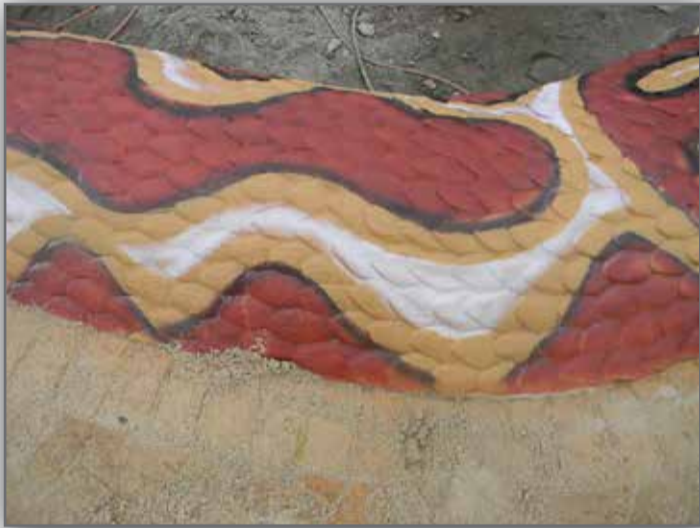
Second Coat of Paint applied - Image 4
